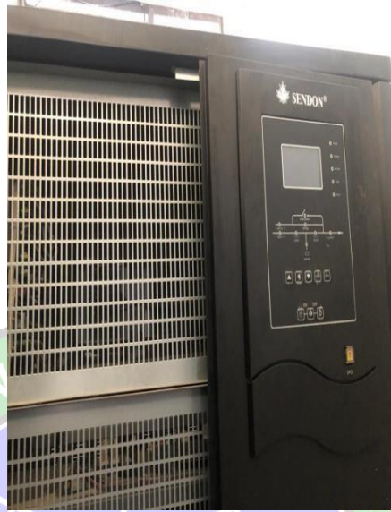
Gambar 4. 3 UPS (Uninterruptible Power Supply)
