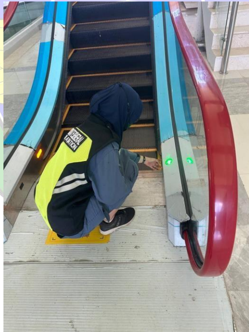
Pengecekan & pengoperasian excalator di terminal baru
