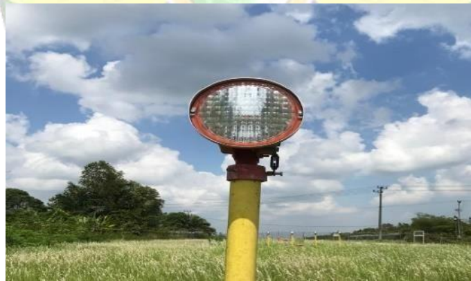
Gambar 2. 6 Approach Lighting System
