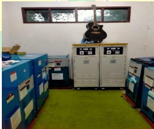
Gambar 2. 28 Constant Current Regulator
