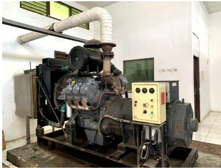
Gambar 2. 30 Generator Set 500 kVA
