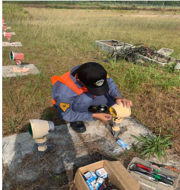
Pergantian Lampu Threshold
