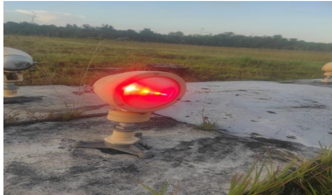
Gambar 2. 11 Runway End Light Elevated
