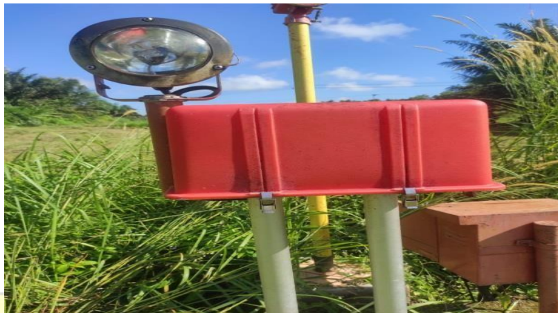
Gambar 2. 19 Sequence Flashing Light
