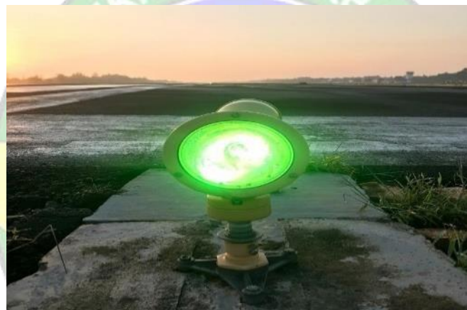
Gambar 2. 8 Lampu Threshold Elevated
