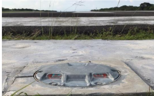
Gambar 2. 7 Lampu Threshold Insert
