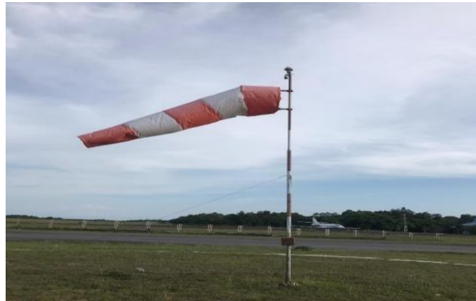
Gambar 2. 17 Wind Directional Indicator Light
