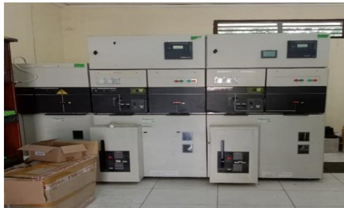
Gambar 2. 25 Panel Cubicle TM
