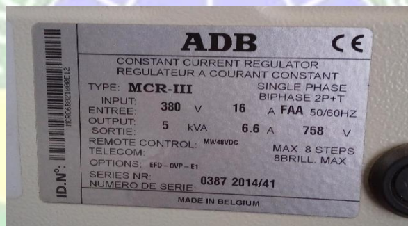
Gambar 2.36CCR Taxiway Edge Light Rangkaian C
