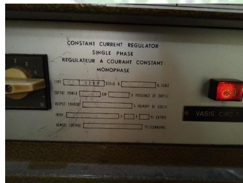
Gambar 2.33 CCR Precision Approach Path Indicator (PAPI) I
