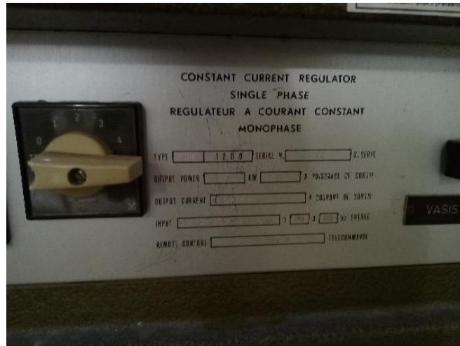
Gambar 2.34CCR Precision Approach Path Indicator (PAPI) II
