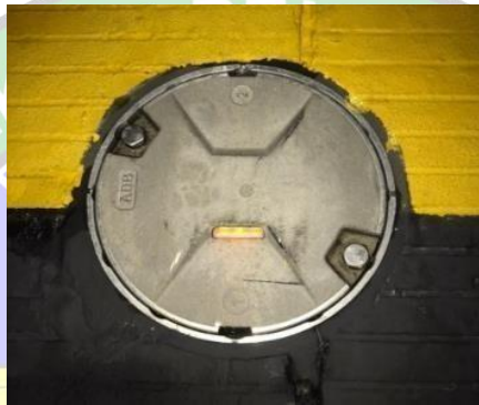
Gambar 2. 12 Rapid Exit Taxiway Light Sumber: Bandar Udara Internasional Yogyakarta
