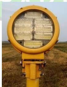
Gambar 2. 3 Sequence Flashing Light
