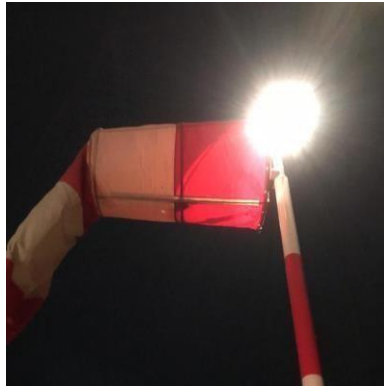
Gambar 2. 14 Wind Direction Indicator/ Wind Cone Sumber: Bandar Udara Internasional Yogyakarta
