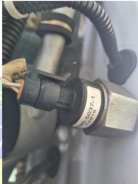
Gambar 4. 2 : Instalation oil pressure tranducer
