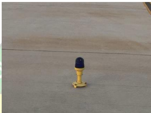
Gambar 2. 18 Turning Pad Light
