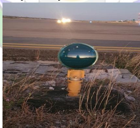
Gambar 2. 17 Wingbar Threshold Light
