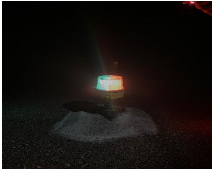
Gambar 2. 15 Threshold Light
