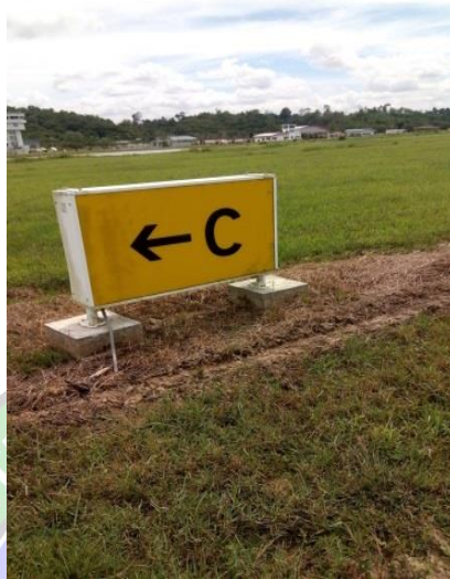
Gambar 2. 33 Taxiway Guidance Sign
