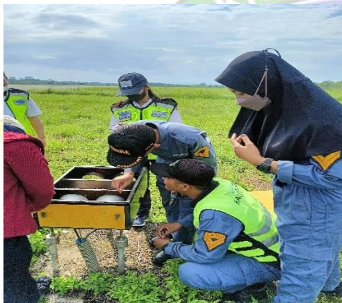
Maintenance Lampu PAPI
