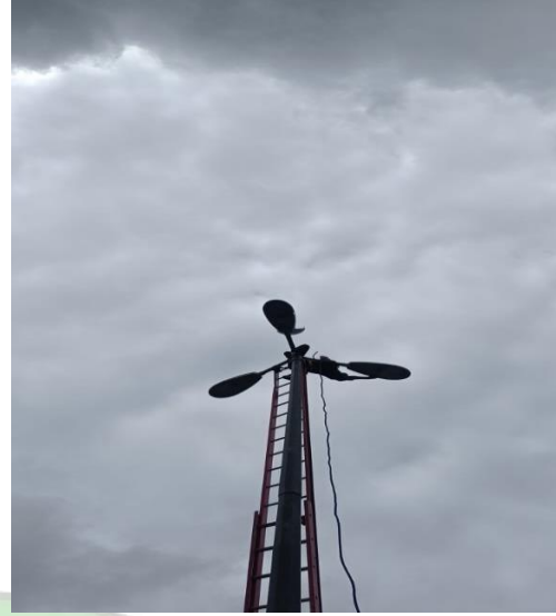
Maintenance Lampu Jalan
