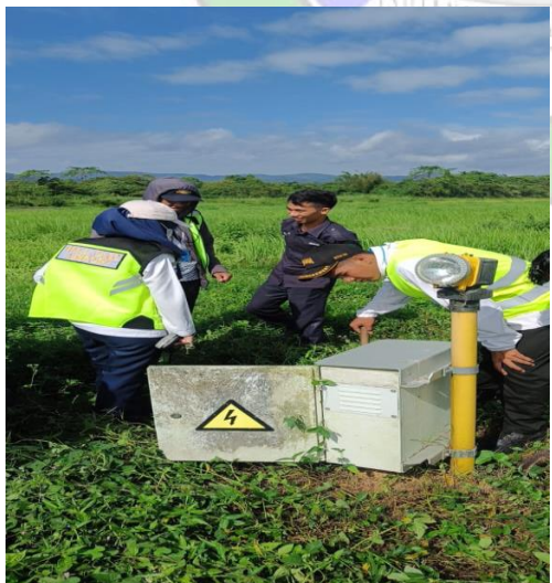
Maintenance Lampu RTIL
