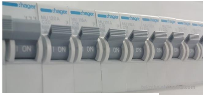
Gambar 3. 9Miniature Circuit Breaker
