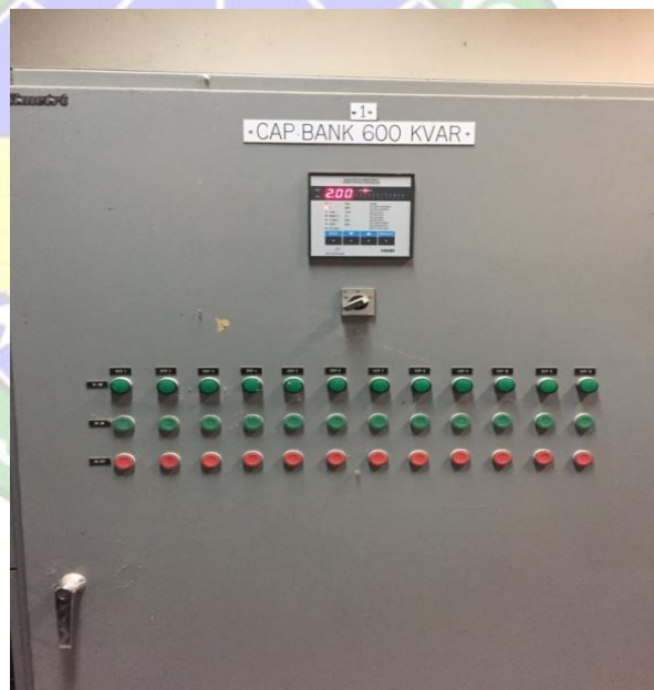
Gambar 4. 10 Capasitor Bank
