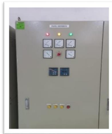
Gambar 4. 8 Out Going Distribution Breaker
