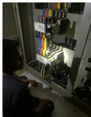
Gambar 4. 36 Switch manual
