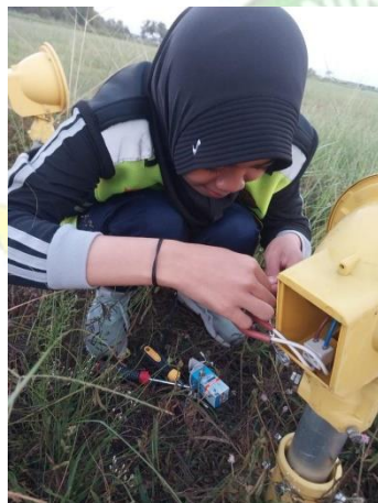
PENGANTIAN BOHLAM APPROACH LIGHT
