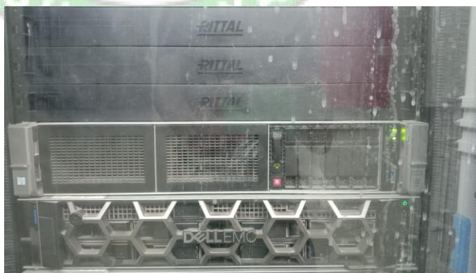
Gambar 3. 1 Server Flight Information Display System (FIDS)
