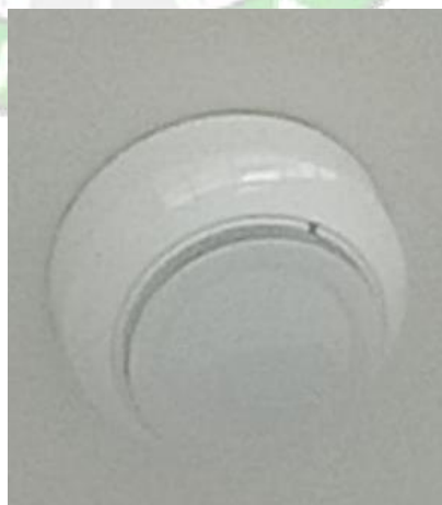
Gambar 3. 4 Smoke Detector
