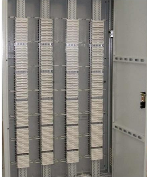
Gambar 3. 20 Panel Main Distribution Frame (MDF)
