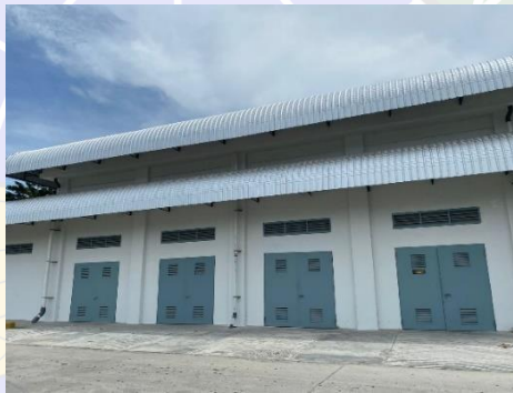
Gambar 4. 7 Gedung Power House
