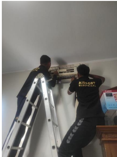
Gambar 9 Pencucian indoor AC
