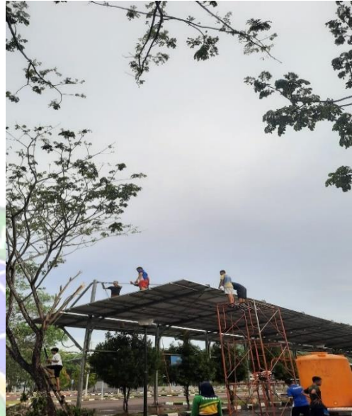
“Pembersihan Solar cell Bandara”
