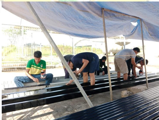
“Pengecatan tiang besi solar cell”
