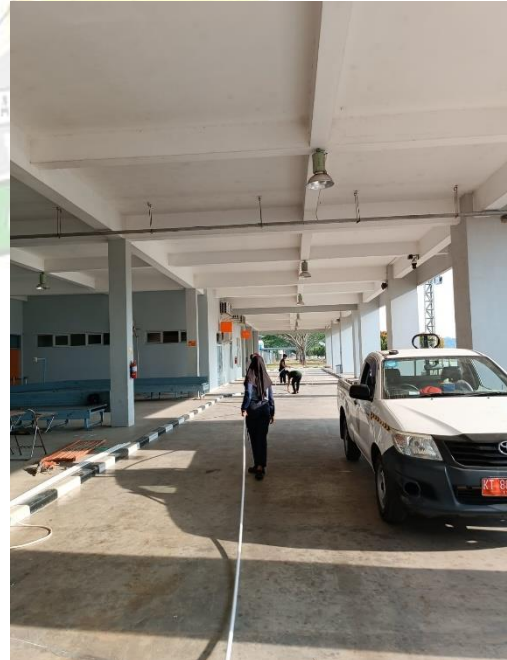
"Pemasangan kabel AC outdoor"
