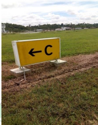
Gambar 2. 33 Taxiway Guidance Sign
