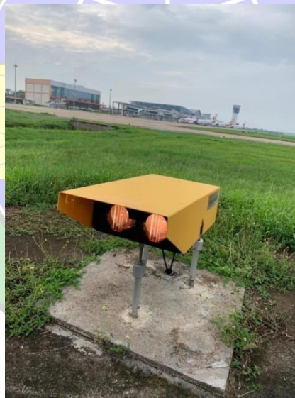
Gambar 2. 9 Precision Approach Path Indicator (PAPI)
