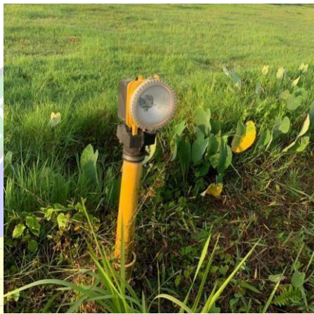
Gambar 2. 3 Sequence Flashing
