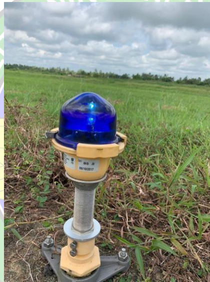
Gambar 2. 11 Turning Area Light
