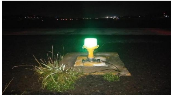
Gambar 2. 5 Threshold Light Elevated Sumber : Bandara Husein Sastranegara
