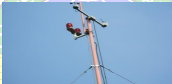
Gambar 2. 21 Obstruction Light Sumber : Bandara Husein Sastranegara
