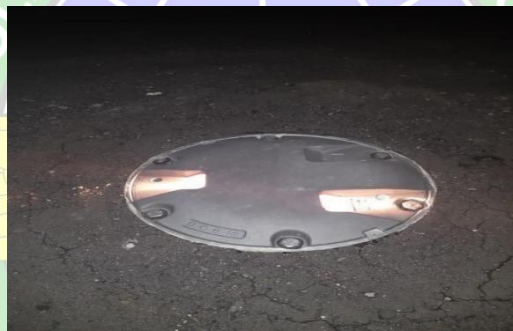
Gambar 2. 8 Runway Edge Light Insert
