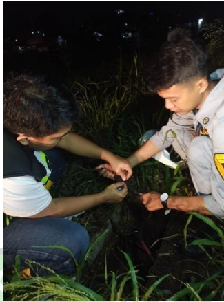
11. Perawatan trafo series
