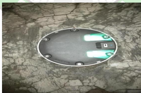
Gambar 2. 6 Threshold Light Insert Sumber : Bandara Husein Sastranegara
