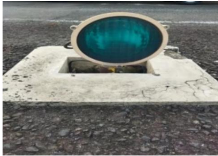
Gambar 2. 14 Wingbar Threshold Light
