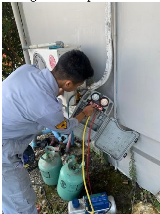
7.Pengecekan Pipa AC Outdoor
