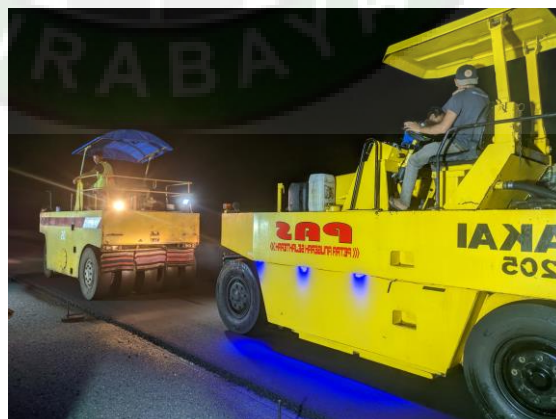
Gambar 4. 22 Pneumatic Tire Roller
