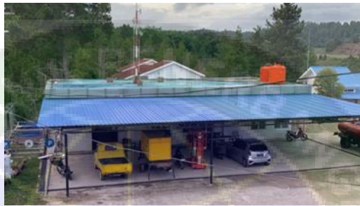
Gambar 4. 8 Gedung Power House
