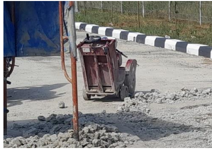
Gambar 4.30 Concrete Cutter Sumber: Olahan Penulis, 2023
