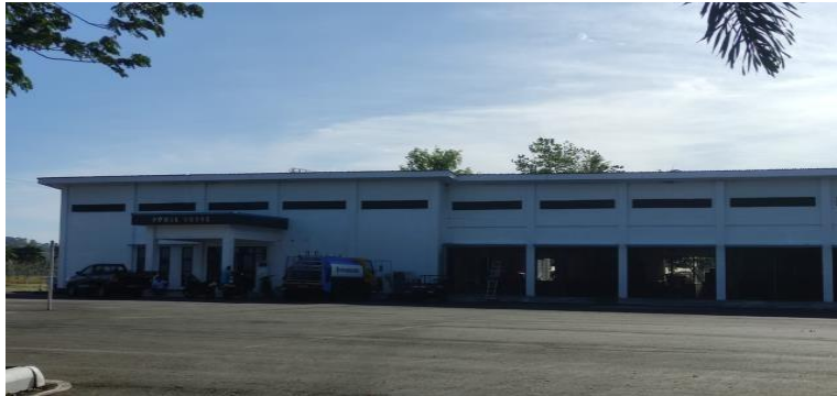
Gambar 4. 10 Gedung Power House
