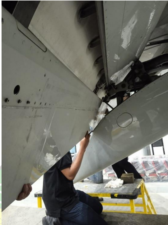
Gambar 4. 9 Flap upper surface install
