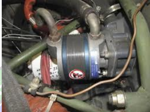
Gambar 4. 7 install vacuum pump
