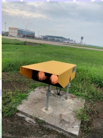
Gambar 2.9 Precision Approach Path Indicator (PAPI)
