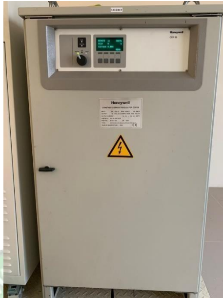
Gambar 3.3 CCR Honeywell
