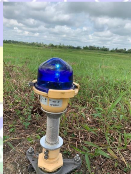
Gambar 2.11 Turning Area Light
