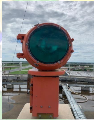
Gambar 2.10 Rotating Beacon Light
