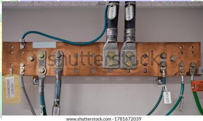
Gambar 3. 13 grounding busbar
