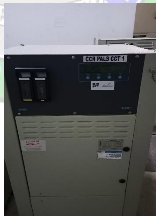
Gambar 2. 29 Constant Current Regulator
