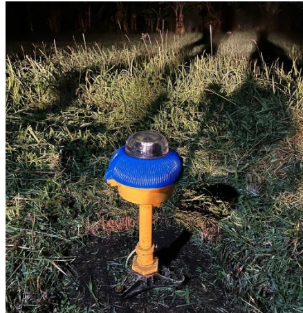
Gambar 2. 18 Turning Area Light
