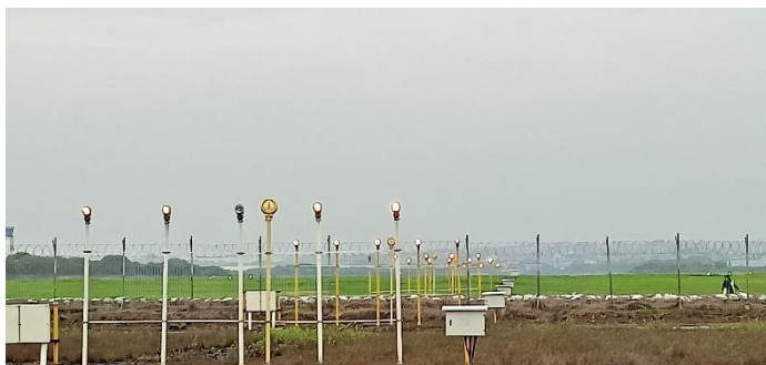
Gambar 2. 13 PALS ( Precision Approach Lighting System ) CAT 1
