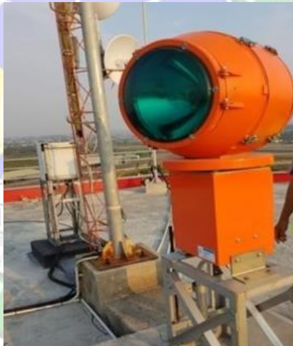
Gambar 2. 19 Rotating Beacon
