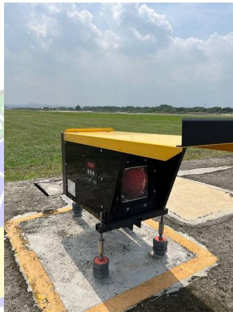
Gambar 2. 15 Precision Approach Path Indicator (PAPI)
