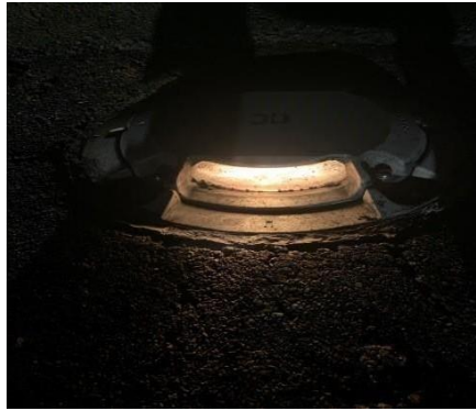
Gambar 4. 5 APPROACH LIGHT INSET
