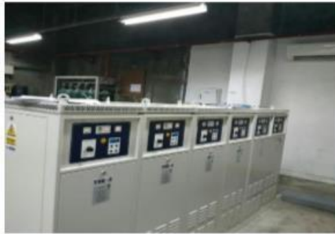
Gambar 4. 3 CONSTANT CURRENT REGULATOR (CCR) DI TI
