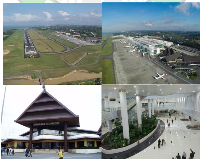
Gambar 2. 3 RUNWAY, APRON SERTA TERMINAL LAMA & TERMINAL BARU
