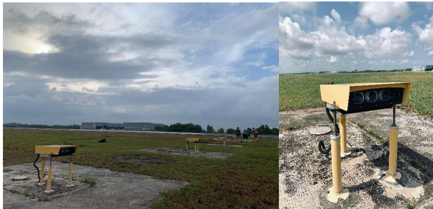
Gambar 3. 2 Precision Approach Path Indicator (PAPI) Sumber : Bandara Internasional Hang Nadim Batam
