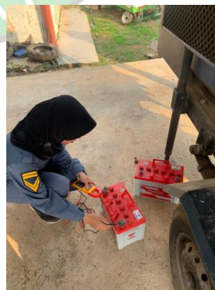
Pengecekan Aki Genset Portable
