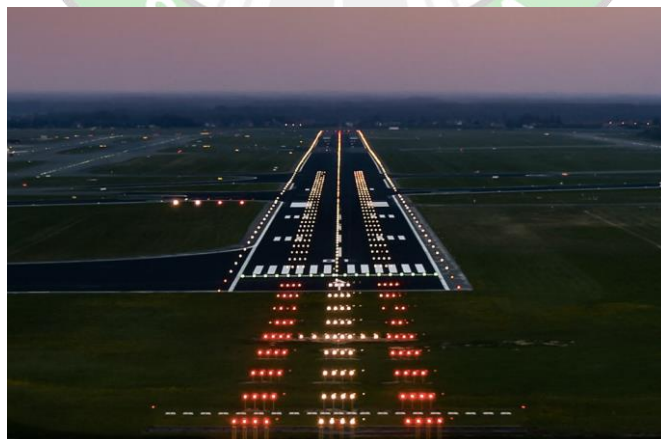
Gambar 3. 1 Airfield Lighting System Sumber : (boldmethod.id)
