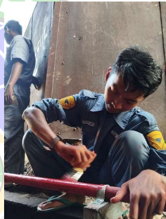
Pengecatan Pipa Bahan Bakar Genset
