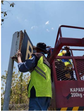
Penggantian Lampu TL Parking Stand
