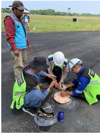
Penggantian Lampu Taxiway Edge Light
