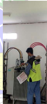
Perawatan Gardu Cargo
