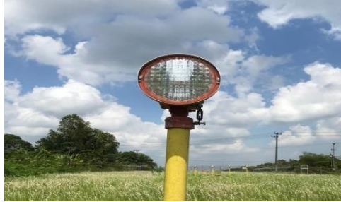
Gambar 2. 7 Approach Lighting System
