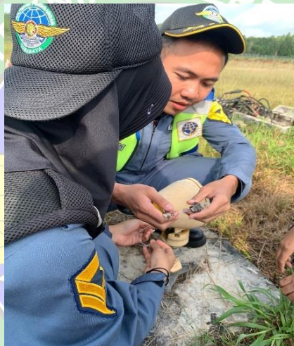
Penggantian Lampu Threshold Elevated
