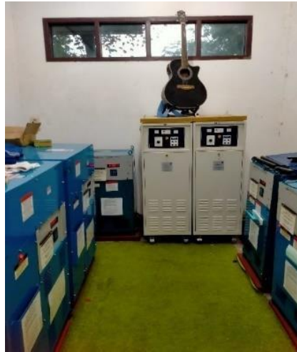
Gambar 2. 29 Constant Current Regulator
