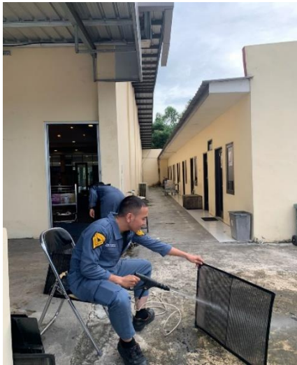
Pencucian Filter AC 5 PK
