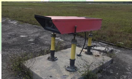
Gambar 2. 6 Precision Approach Path Indicator (PAPI)
