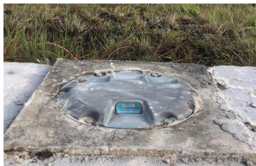
Gambar 2. 11 Runway End Light Insert
