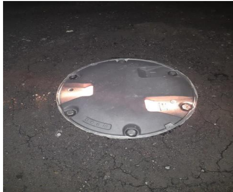
Gambar 2. 5 Runway Edge Light Insert
