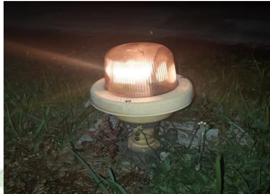
Gambar 2. 4 R/W Edge Light Elevated
