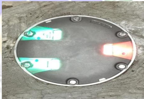
Gambar 2. 8 Lampu Runway End (Insert)
