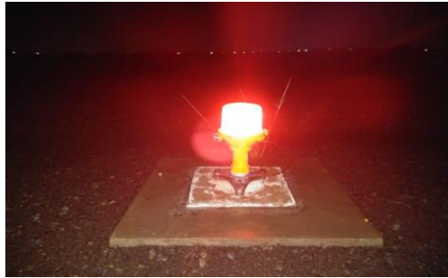
Gambar 2. 9 Runway End Light Elevated Sumber : Bandara Internasional Husein Sastranegara
