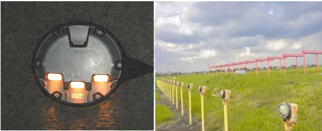
Gambar 2. 8 Approach Lighting System Sumber: Penulis
