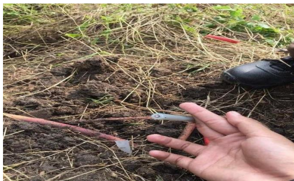
Gambar 4. 10 Pengupasan Outer Sheat Kabel FL2XCY
