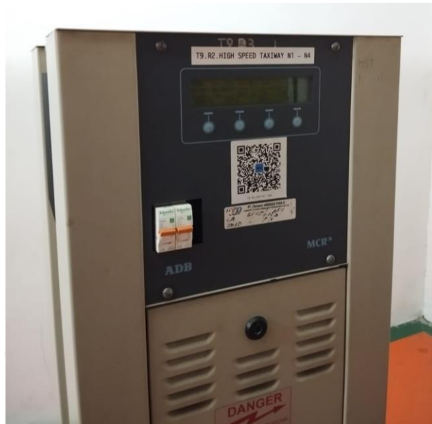
Gambar 2. 27 Constant Current Regulator (CCR) Sumber: Penulis
