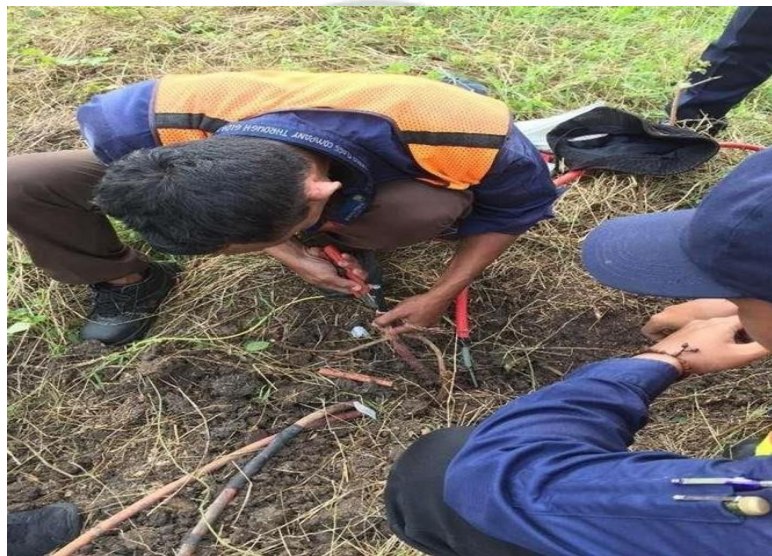
Gambar 4. 11 Proses Cramping Kabel
