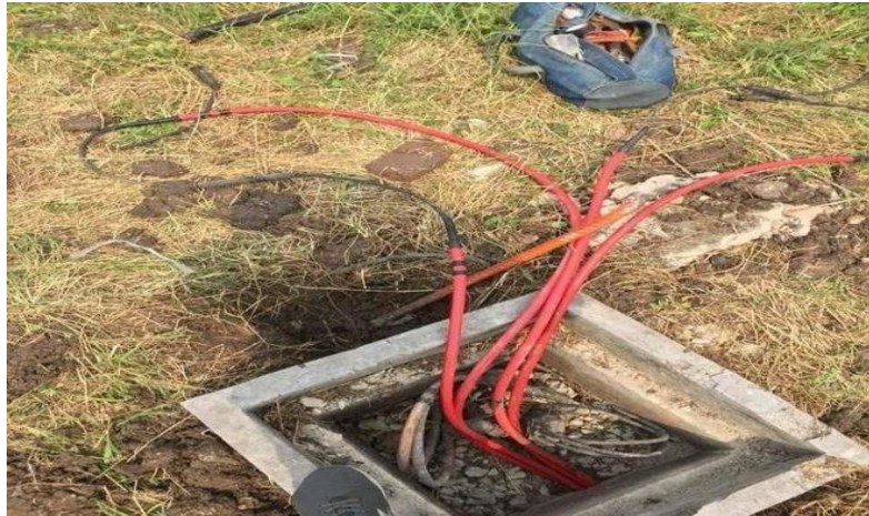
Gambar 4. 12 Penggantian primary connector kit selesai
