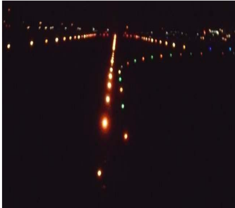
Gambar 2. 14 Exit Taxiway Centerline Light Sumber: Penulis
