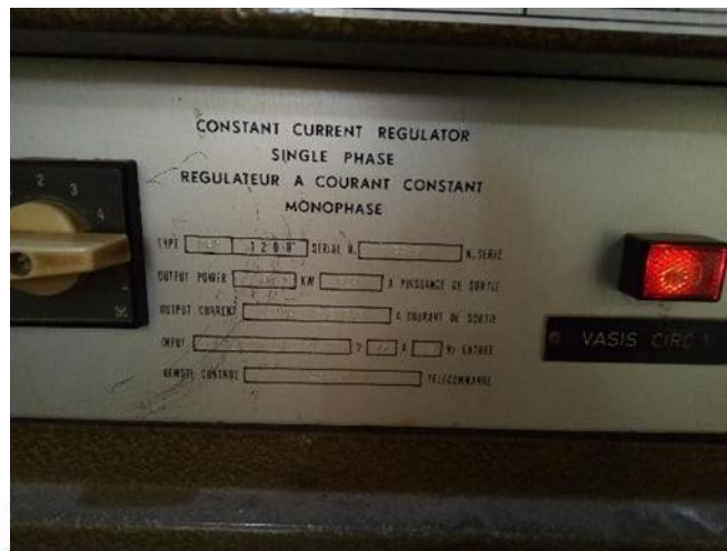
Gambar 2.33 CCR Precision Approach Path Indicator (PAPI) I
