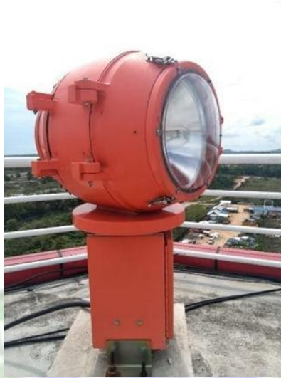
Gambar 2.27 Rotating Beacon
