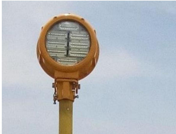
Gambar 2. 21 Runway Threshold Idetification Light (RTIL)
