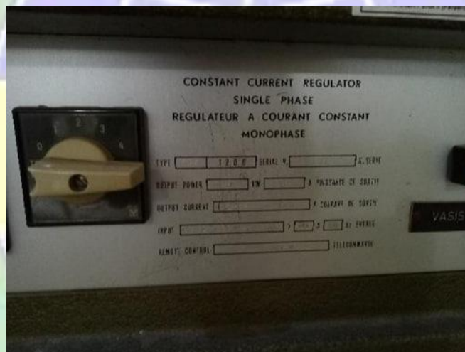
Gambar 2.34 CCR Precision Approach Path Indicator (PAPI) II
