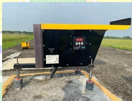
Gambar 2. 17 Precision Approach Path Indicator (PAPI)
