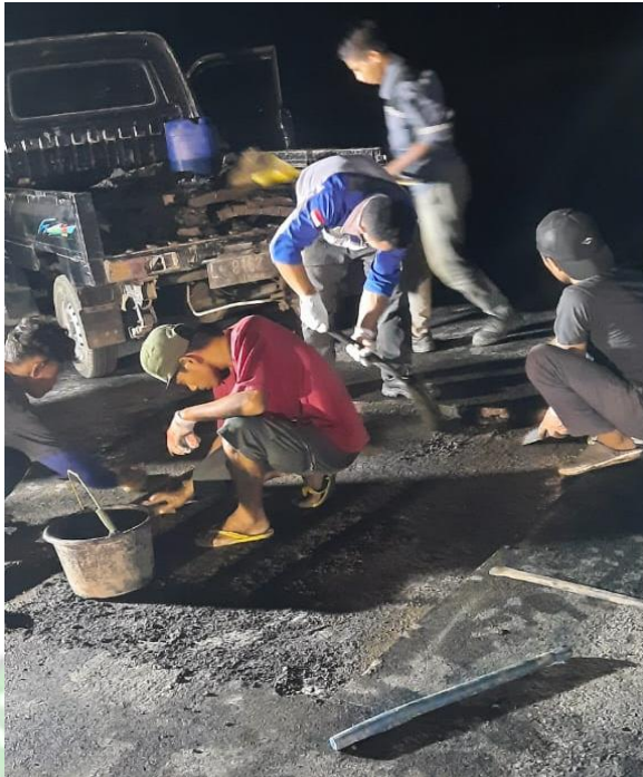
Gambar 4.16 Pembersihan lokasi penambalan ( Patching )
