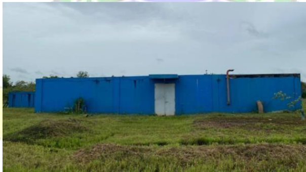
Gambar 4. 16. Water Treatment Plant (WTP) (Sumber : Dokumentasi Penulis, 2024)
