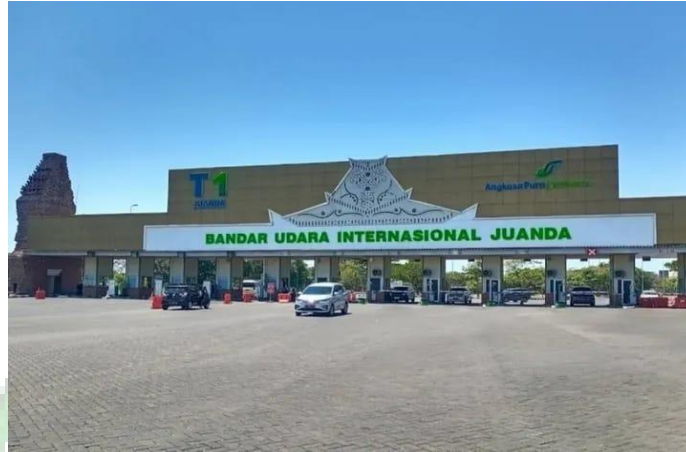
Gambar 2.1 Gerbang Terminal 1 Bandara Internasional Juanda Surabaya
