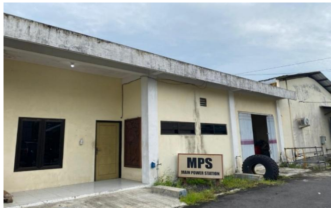
Gambar 4. 9 Gedung Power House
