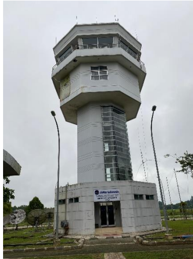
Gambar 4. 9 Menara Air Traffic Controller (ATC)
