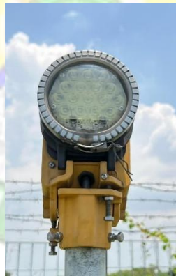
Gambar 3. 1 Lampu Approach Light
