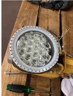
Gambar 4. 4 Ganti Led Approach Light
