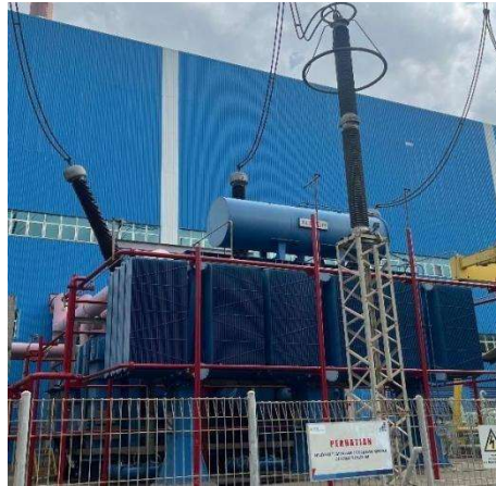
Gambar 3.7 Generator Transformer
