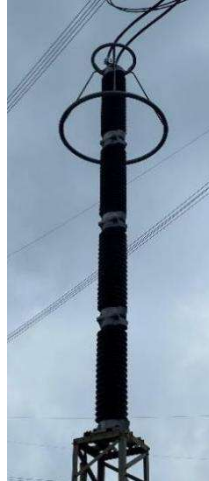
Gambar 3.13 Bushing Trafo
