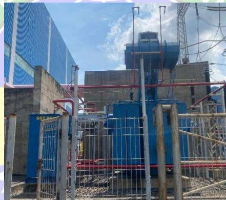
Gambar 3.8 Station service Transformer
